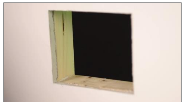
Single plasterboard wall with wooden frame.
